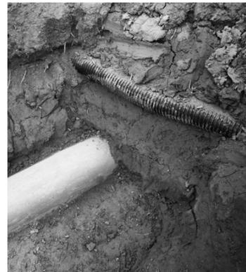
*Cross at an angle as close to 90 degrees as possible and with at least 24 inches of separation.
